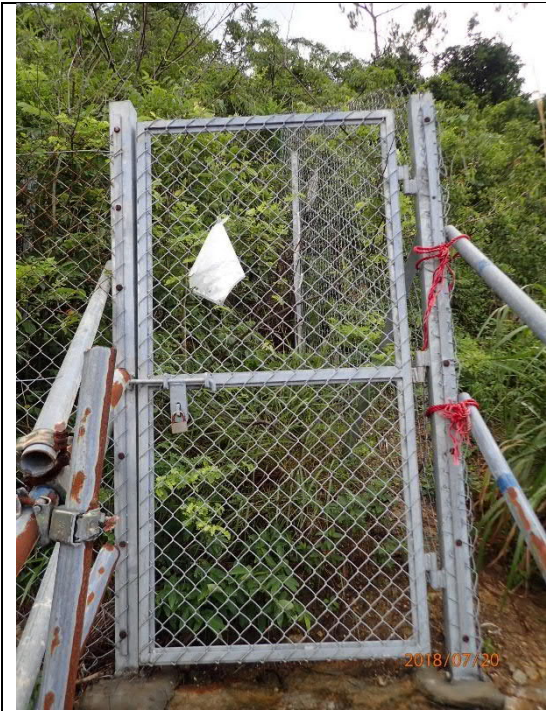
Photo 3 – Current situation of fencing and warning sign
